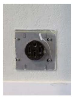
The exterior receptacles are in fairly good working order; however, not all of these receptacles have ground fault protection. Some receptacles are covered with plant growth and need to be cleared out.
