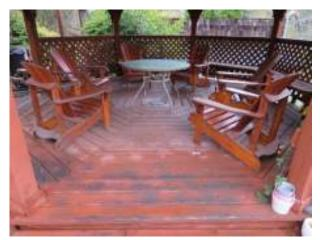
One of the gazebos has wood framed lattice guardrails which do not meet todays' building standards with no climable horizontal guardrails or lattice panels and should be changed to provide sufficient safety.
