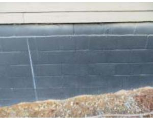
The buildings structural concrete block walls remain in fairly good condition with only minor effloresce seen on some areas due to moisture seepage through the concrete over the years. These areas need to be cleaned up and repainted with a waterproof elastomeric type of paint.
