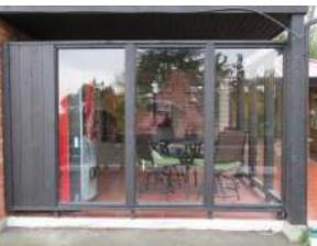
The building has a framed in patio by the lobby with floor to ceiling glass shear walls that do not appear to be tempered glass panels and all need to be reviewed and replaced, as necessary.
