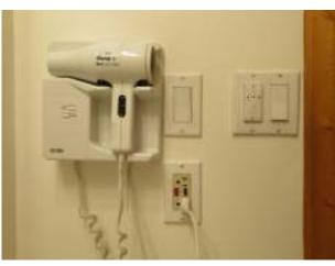
The electrical receptacles tested are operational and in fairly good condition with typical deterioration. All bathrooms inspected have GFCI receptacles installed.
