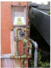
The motel has contracted propane tanks providing fuel for the commercial dryer in the laundry room and they have no visible damage. There is also two tanks located by the gazebos that provide fuel to barbeques on the patio and they are slightly overgrown by plants but also have no visible damage.
