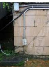
The concrete block retaining walls are in fair to fairly good condition with a few damaged blocks to be repaired along with some moss growth to be removed off the mortar joints and the mortar to be repointed where necessary.
