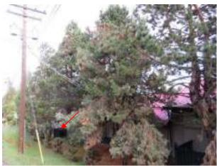
The overhead electric service for the motel has the conductors running though tree branches that need to be professionally cut back to ensure no damage or outages.
