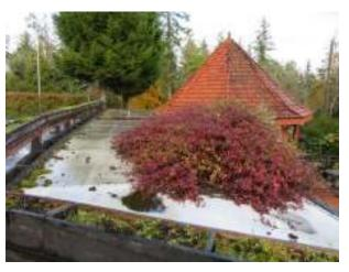
The north end of the patio has an elevated wood framed walkway with a set of wood framed stairs leading down to the lower yard and they are in reasonable to fair condition with handrails that do not meet todays' building standards and have missing planks on the walkway to be replaced as soon as possible to eliminate various trip hazards.
