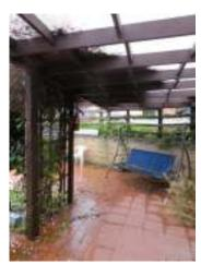
The lower patio has a wood framed pergola with a clear plastic roof cover that is in poor to fair condition with plant overgrowth to be cut back and removed and there are some broken and missing roofing panels to be replaced as well as some minor wood damage to be reviewed and repaired as necessary. There are built-in wood planter boxes around the top of the pergola that are not lined, and the wet soil has deteriorated some of the planters and replacement is required.
