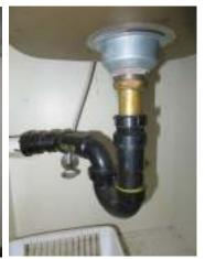
The laundry room sink drainage has an improper 'S" drain trap and leads across the floor to a floor drain and needs to be reviewed and corrected by a licensed plumber to provide proper drainage for the sink, or have the sink removed.
