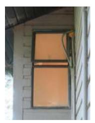
There is one replaced window poorly installed with the window flange and fasteners exposed and needs to be sealed and finished with a wood trim.
