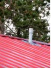
The penetrations through the roof include the skylights, and mechanical venting. Overall, the roof penetrations were noted to be in fair to fairly good condition, some minor repairs and updating of maintenance is required sealing over rising fasteners and replacing them where necessary. No leaks were noted around the roof penetrations on the day of the inspection.
