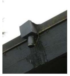
The visible downpipes are in fair condition with some minor dents and damage and some unusual pipe installation to be
