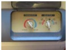
The main building and outer building have various aged wall mounted electric baseboard heaters that are in fairly good condition with only some minor dents and slight damage to a few here and there. The baseboard in the north outer building has wood products stored up against it and the heater needs to be cleared of any contact with combustibles.
